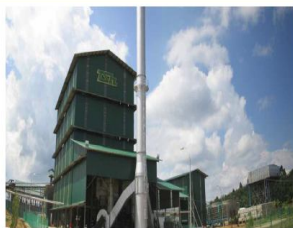
Figure 9: Janal Landfilbiogas power plant
